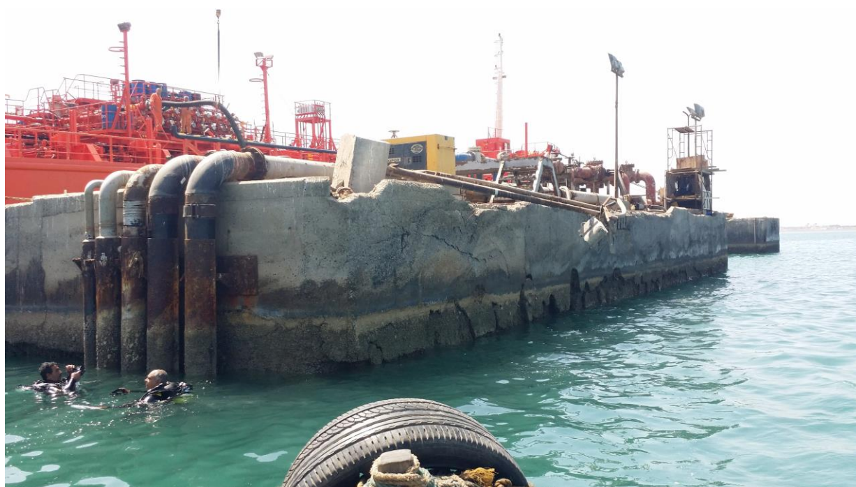
Photo : UNDP Yemen. Port of Hodeidah.
