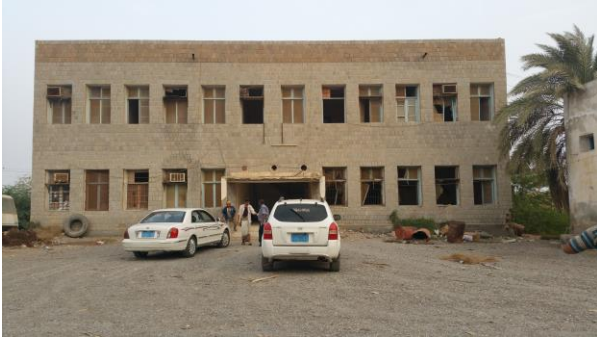
Photo: Port of Hodeidah Training Center prior to rehabilitation. UNDP
