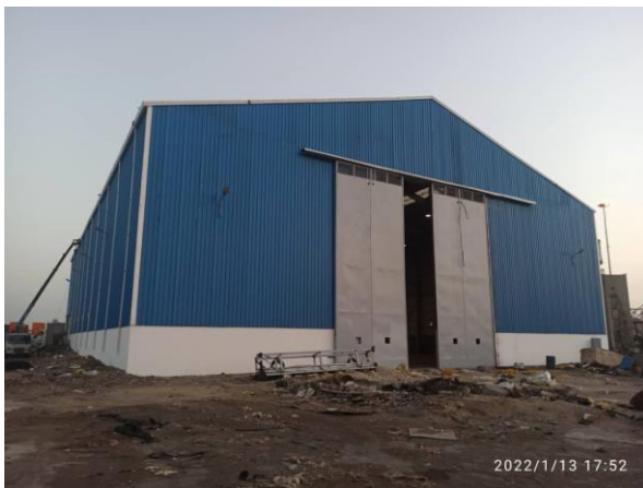
Photo: Maintenance workshop after
