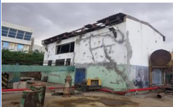
Photo: Slipway facility before rehabilitation.UNDP
