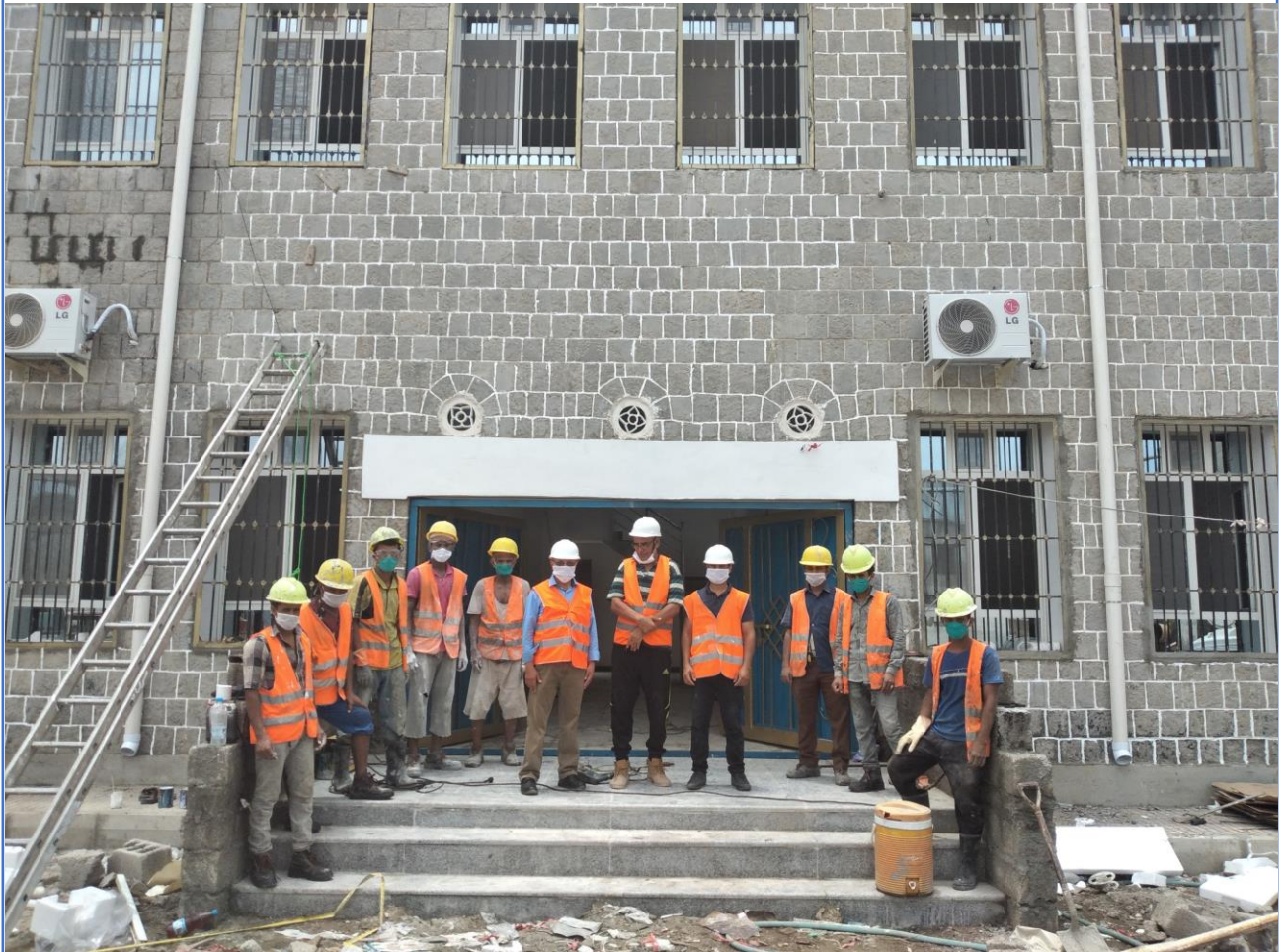
Photo: Construction workers rehabilitating the Training Center in Port of Hodeidah
