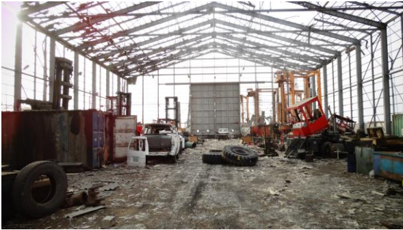
Photo: Maintenance workshop before
