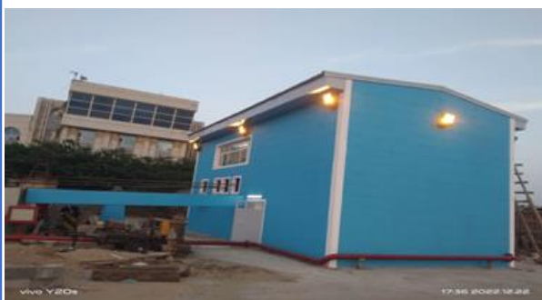
Photo: Slipway facility after rehabilitation.UNDP
